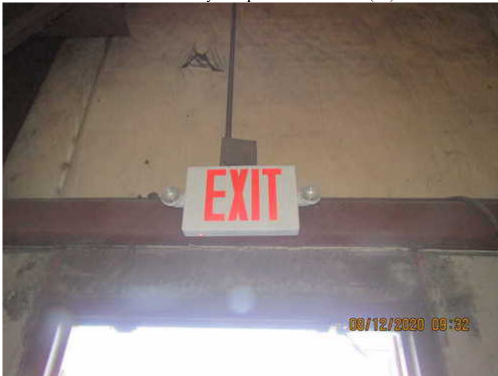
5770 N Industrial Pkwy - Inspection 8-12-2020 (44).JPG
